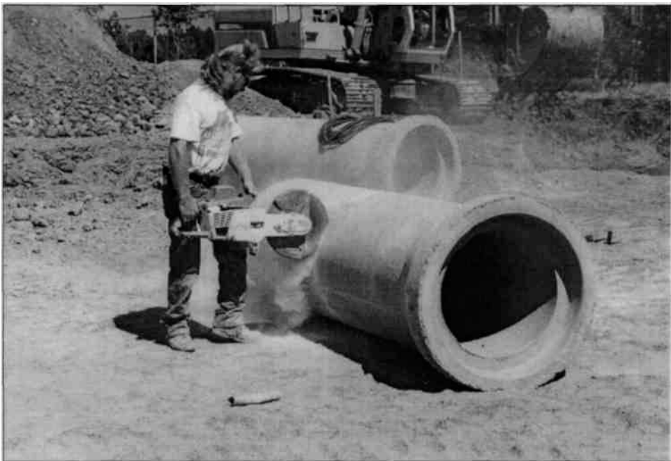
The saw is cutting through a 2 foot diameter concrete drainage pipe.
